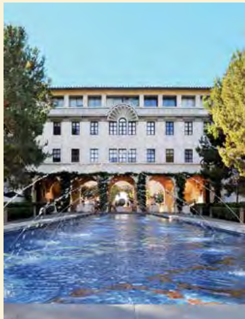
Caltech's Beckman Institute is a multi-disciplinary research center for the chemical and biological sciences.
