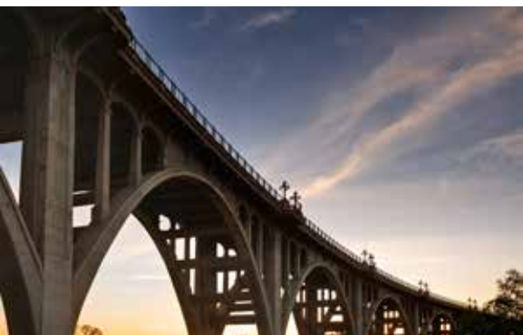
Colorado Street Bridge
